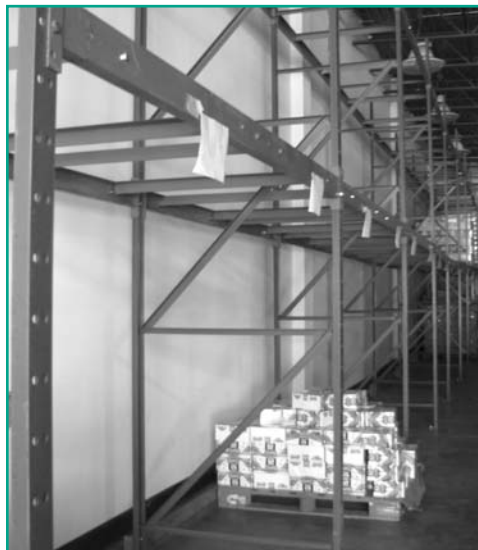
Empty racks which previously contained pallets of USDA commodities
